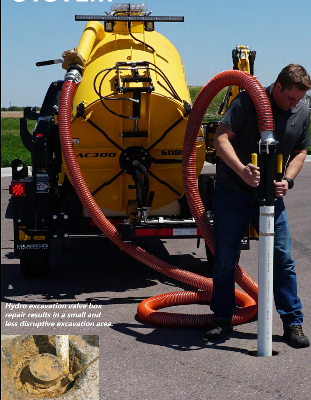
Hydro excavation valve box repair results in a small and less disruptive excavation area.
